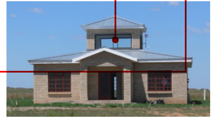
Figure 1.12 Air Traffic Control Tower. (Karihindi, 2015)
