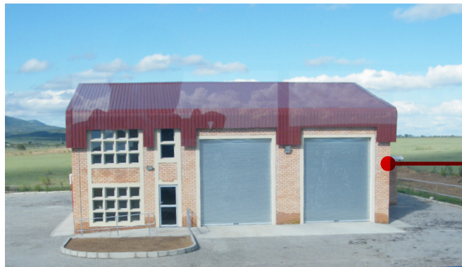
Figure 1.11 New Fire Station. (Karihindi, 2015)
