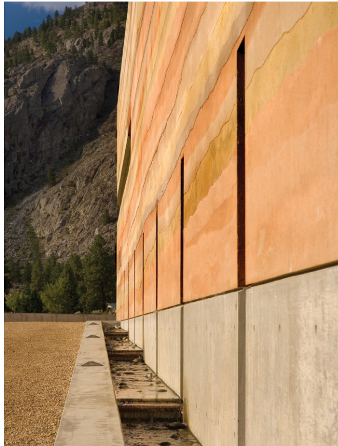
Figure 8.8 Structural Insulated Rammed Earth. (n.d.)
