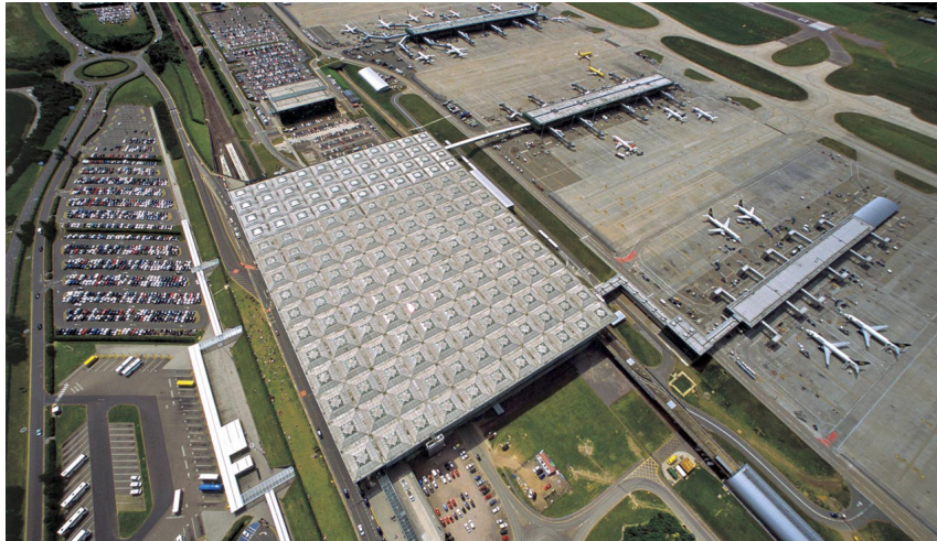
Figure 7.0 Aerial photograph showing terminal with adjacent apron. (Foster and Partners, 2009)
