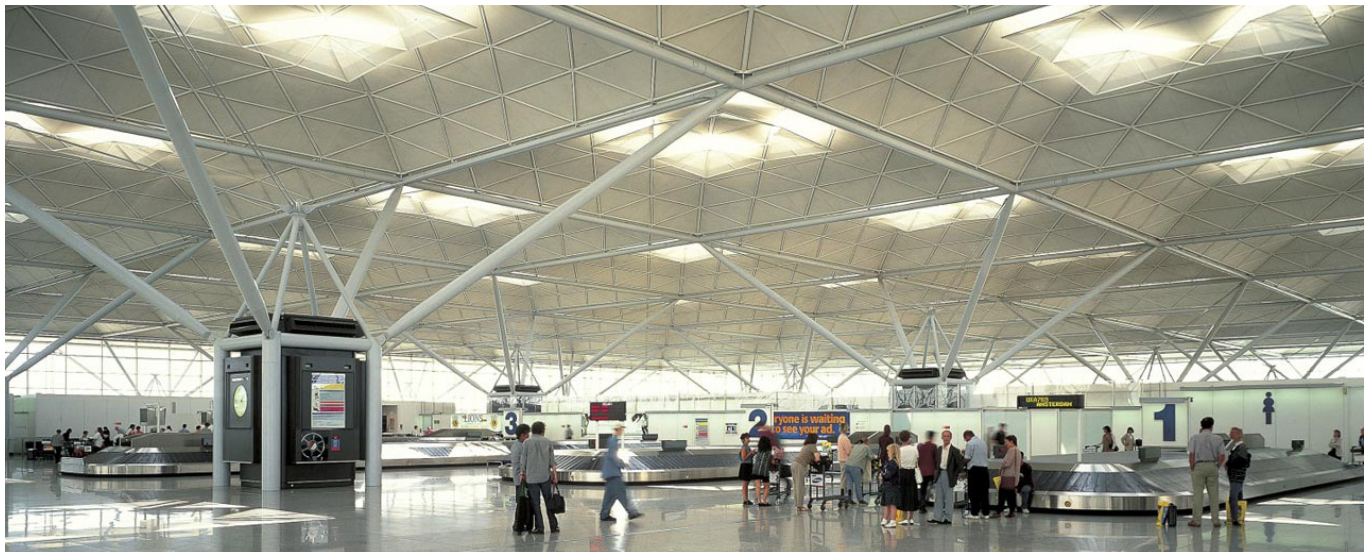
Figure 7.1 Baggage reclaim Hall. (Foster and Partners, 1991)
