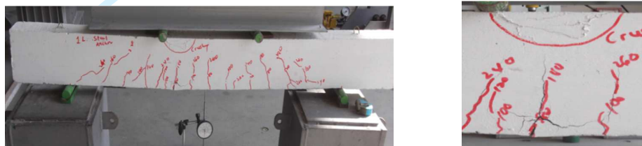
(a) Rupture of GFRP with concrete crushing failure of beam FSB-SA1
