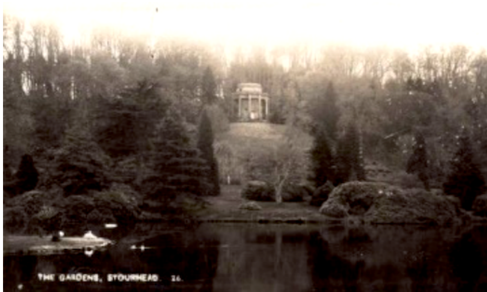
Figure 4.1 – Early nineteenth-century postcard published by Frederick Holmes showing Temple of Apollo in a state of disrepair
