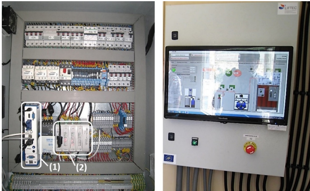
Figure 4. Inside (left) and outside (right) images of the main control cabinet
