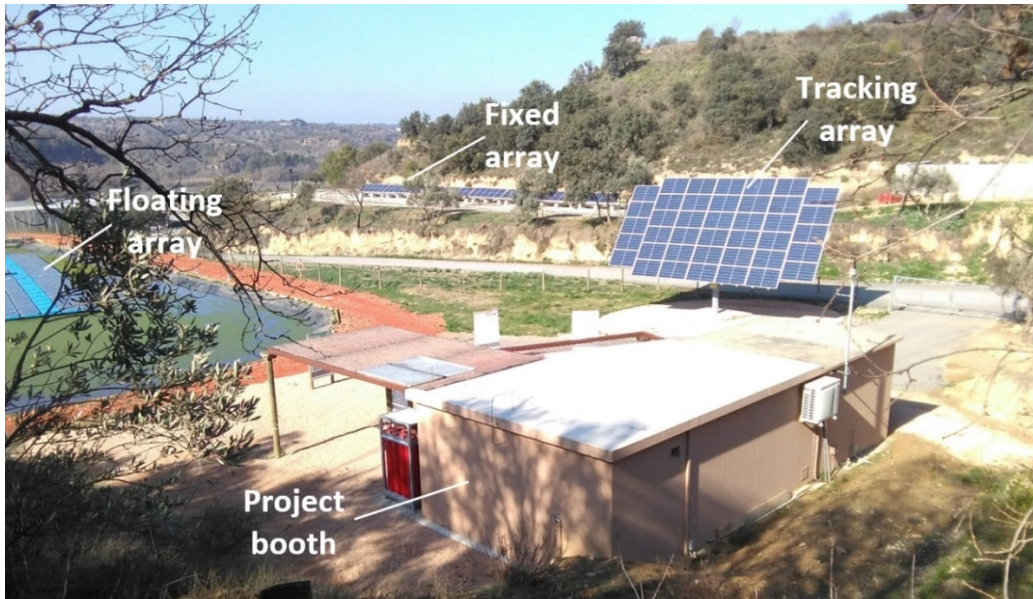
Figure 3. Assembling of the different solar arrays and main project booth at the
