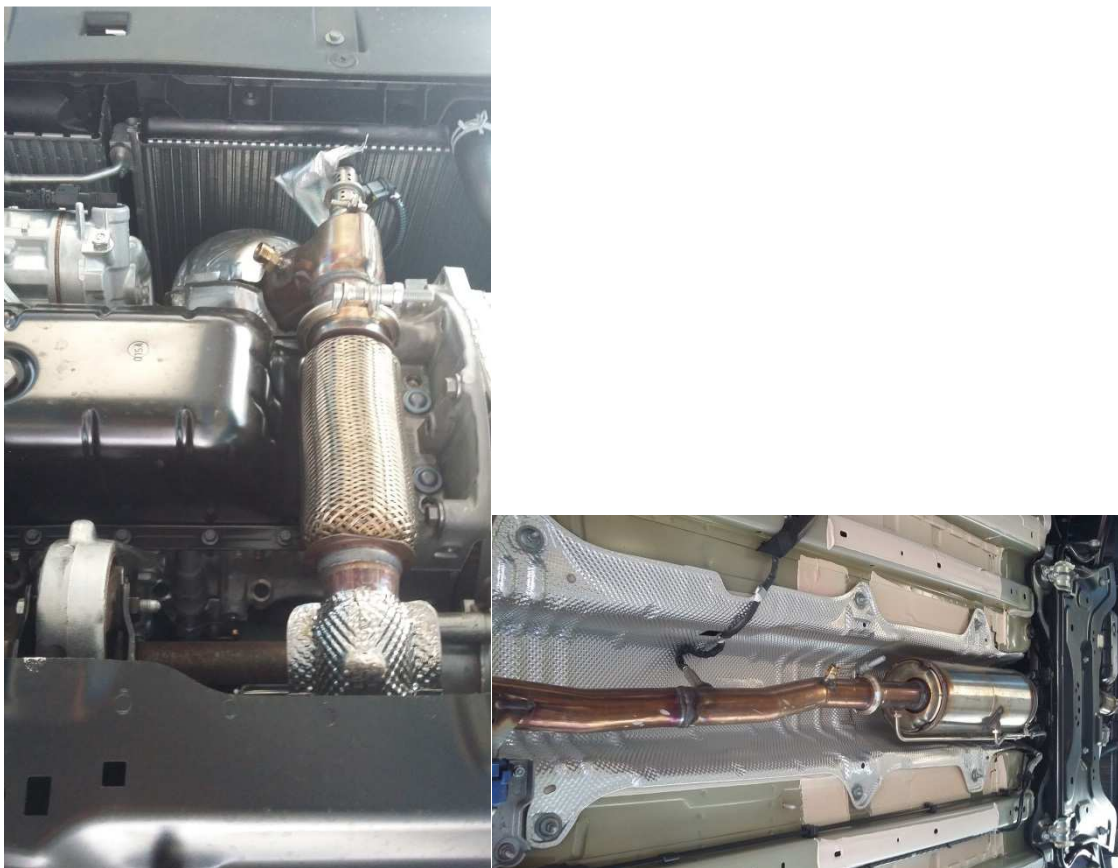
Figure 31. Installation of the pre-cat thermocouple close to the lambda sensor (left panel) and post-cat thermocouple under-floor (right panel) for the measurement of the temperatures before and after the after-treatment system.
