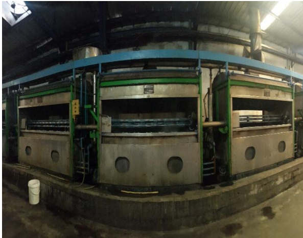
Figure 3.20. Re-washing and Re-drying Machine
