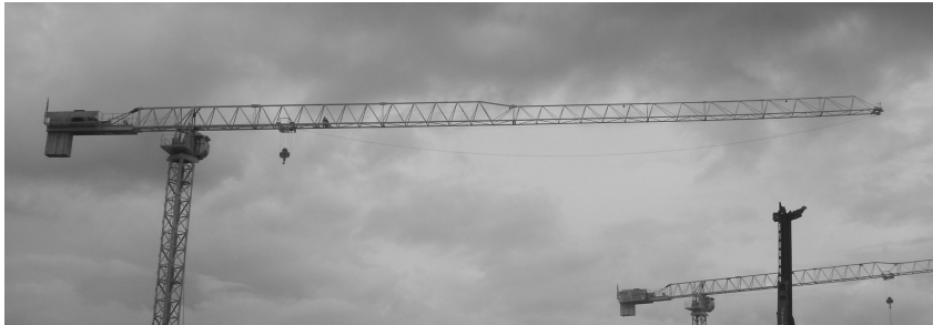
Figure 1: Picture of the crane in the construction yard.
