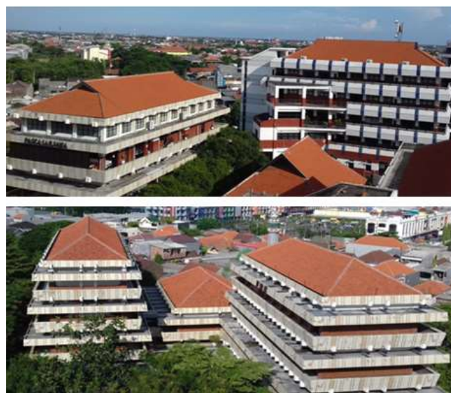
Fig. 2. Gablet roof (upper) and Hip roof (lower) types buildings at of University of Surabaya
