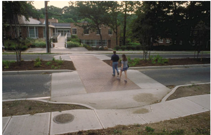
Figure 3: A raised crosswalk with differentiated pavers, along with a raised centre median / pedestrian refuge island.
