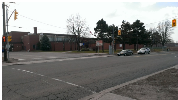
Figure 9: West Hill Collegiate, view from main entrance at Morningside Avenue.
