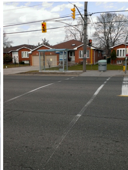
Figure 22: Pedestrian crossing in front of WHCI, and northbound bus shelter.
