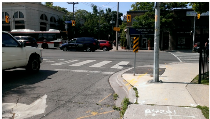
Figure 4: A curb extension narrows the roadway, allowing for shorter crossing distances as well as calming traffic.
