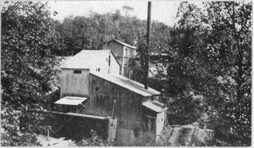
A.—Clay mill of the Ceramic Clay Company, Pedro. (Photo by C. E. Bales.)
