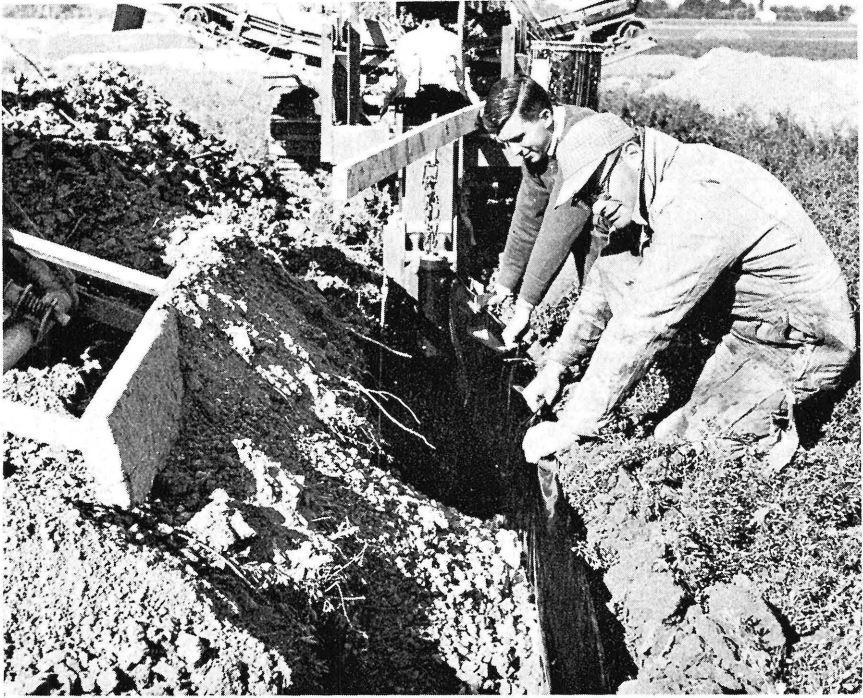
Fig. 3.—Installation of plastic barrier.
