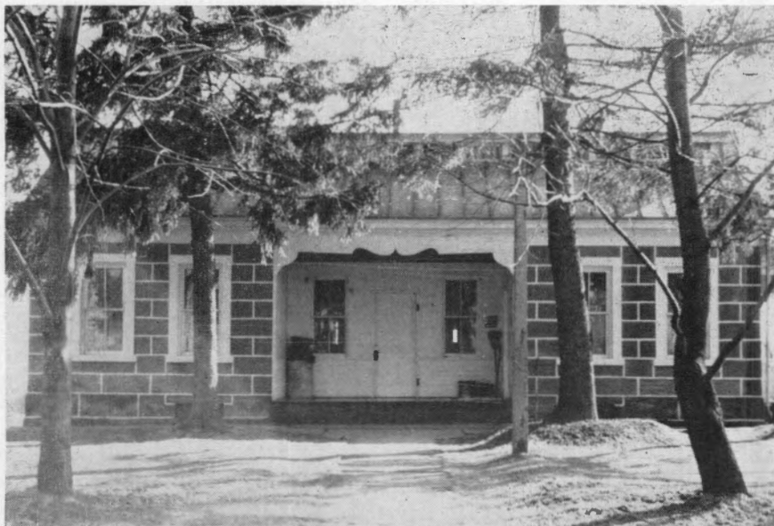
FIGURE 8. View of Wm. Kindleberger's house, constructed from a high Greene series sandstone.
