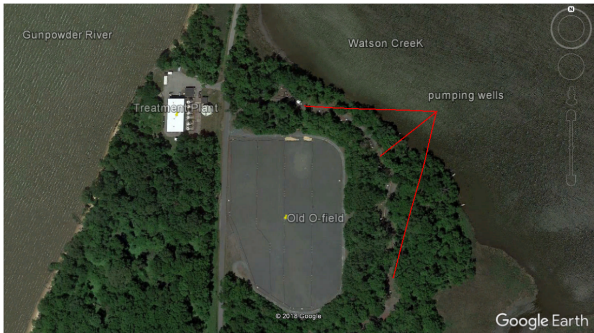
Figure12. This figure from Google Earth shows the Old O-Field area, the pumping wells for the remediation system and the treatment facility. Major water bodies shown are Watson Creek and Gunpowder River. The photo was taken on 5/25/2013.
