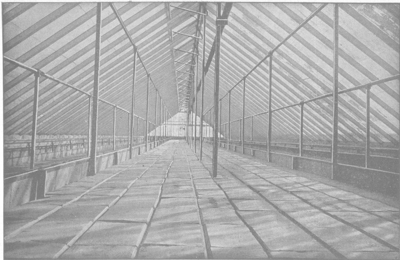
FIG. II.—INTERIOR OF GREENHOUSE, SHOWING TILE BOTTOMS AND SLATE SIDES TO BENCHES.
