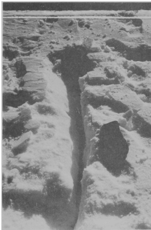
Fig. 17 - Crack 7 cm wide on the surface at Mile 285. Mitten to right of crack (Photo by R. L. Cameron)
