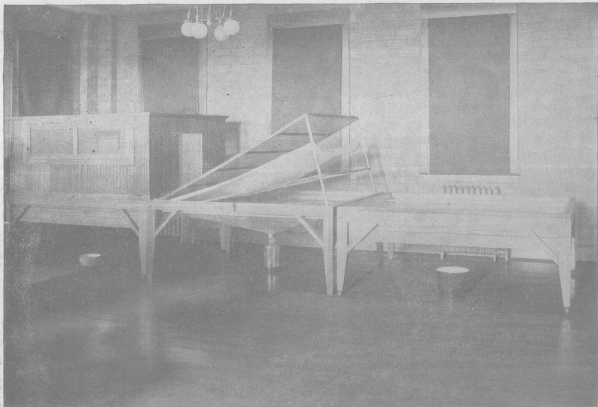
PLATE II Metabolism crate—Top removed, screens and cloth elevated.
