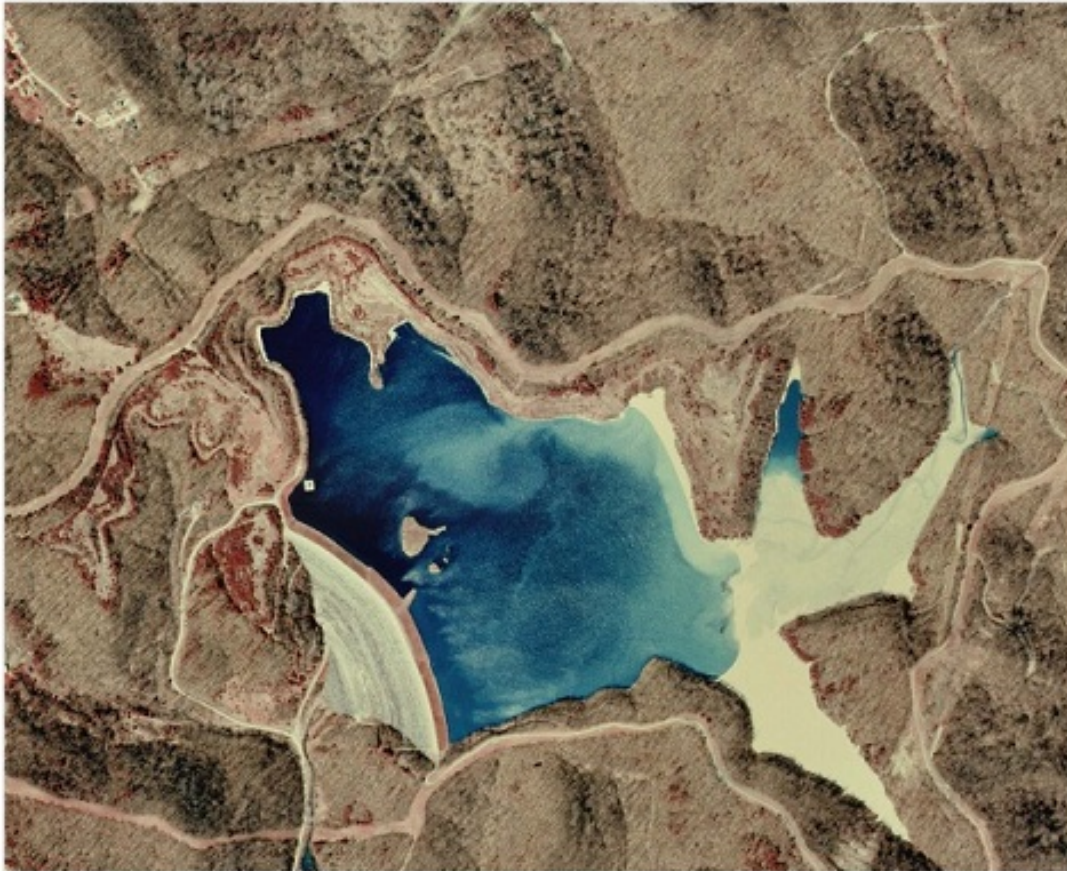
Figure 1:An aerial photo of a fly ash pond (EPRI)
