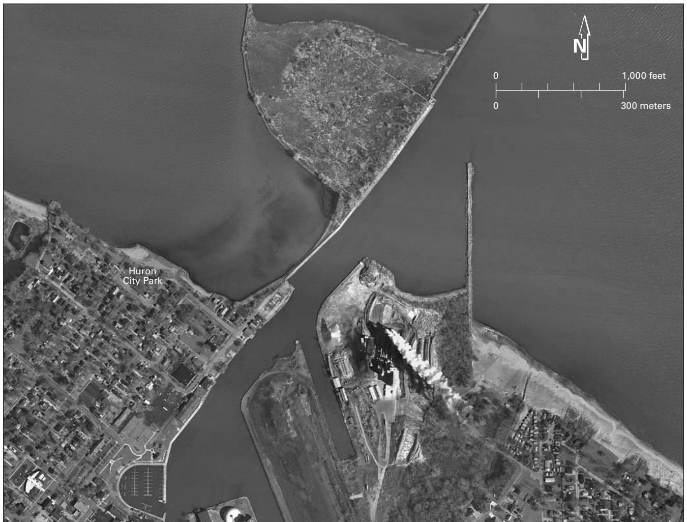
FIGURE 44.—Nickel Plate Beach to the east of Huron Harbor and Huron City Park to the west, in Huron, Ohio. The beach at the city park is protected by a sandstone breakwater. Steam and smoke from the limekiln make a prominent landmark for boaters. Aerial photograph taken in 2003 by the Erie County Auditor.
