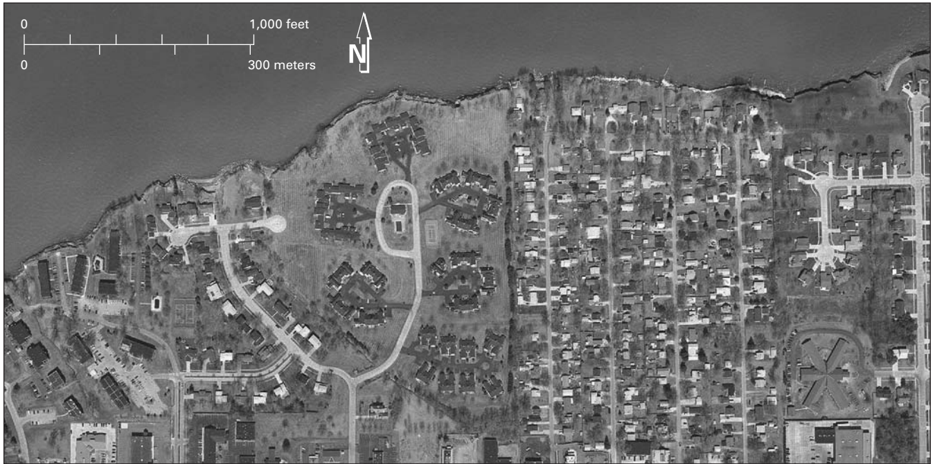
FIGURE 37.—Fault-controlled erosional embayments along the shale-bluffed shore in Vermilion, Ohio (1999). See figure 38 for orientation of faults. Aerial photograph taken in 1999 by the Lorain County Auditor.
