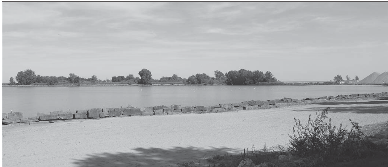
FIGURE 45.—View from Huron City Park, Huron, Ohio, looking lakeward across the beach and a sandstone-block breakwater at a CDF built to contain contaminated sediment dredged from Huron Harbor. Trees are growing on sediment placed in the facility. To the right are piles of limestone brought in by ship for use in a local lime plant. Photograph taken by Laura J. Moore.
