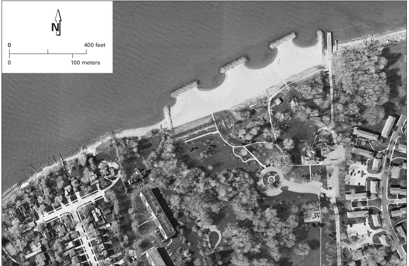
FIGURE 27.—Segmented breakwaters and terminal groins at Sims Park in Euclid, Ohio. The breakwaters are spaced so that tomboles develop. The beach was filled with sand obtained from an upland sand pit. Aerial photograph taken in 2002 by the Cuyahoga County Engineer.
