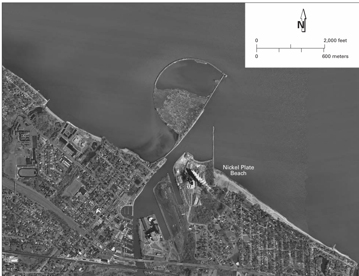
FIGURE 43.—The west jetty at Huron Harbor, Huron, Ohio, extends about 3,410-ft (1,039-m) offshore, blocking littoral transport of sand. A wide beach of sand impounded by the east breakwater extends about 3,300 ft (1,000 m) and is wide enough to support dune development. Beaches west of the harbor tend to be very narrow and seawalls are needed to prevent erosion of the low bank. Aerial photograph taken in 2003 by the Erie County Auditor.
