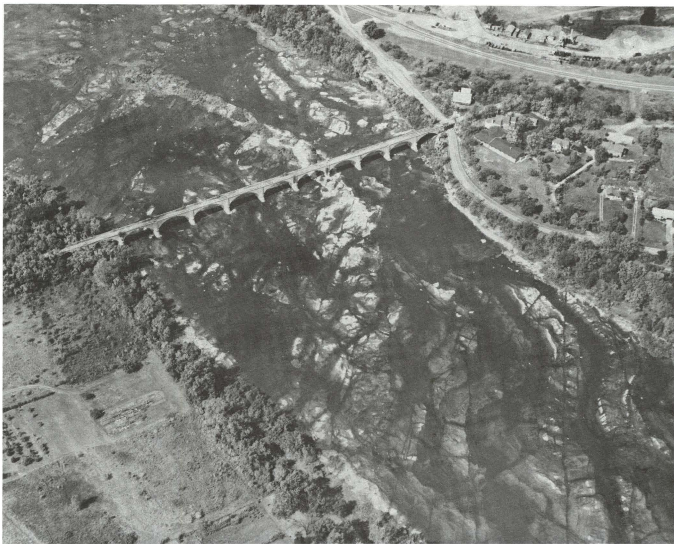
FIGURE 27.—Aerial photograph taken during drought of 1934 showing fault and fracture traces in the bed of the Maumee River along the Bowling Green Fault Zone. Southern edge of the France Stone Co. Waterville quarry is in upper right of photo. Forst Road bridge over the river is oriented N-S. Photo courtesy of the Ohio Historical Society.
