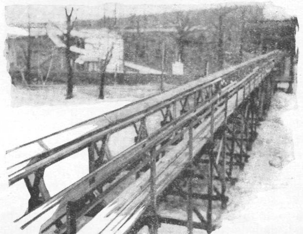
Rubber-Lined Gutters in Which the Nitroglycerin Flows to the Storehouse
