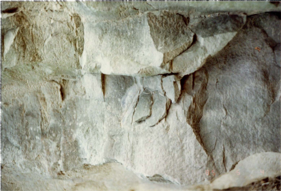
Photo 6. Close up of the sandstone in photo 5.
