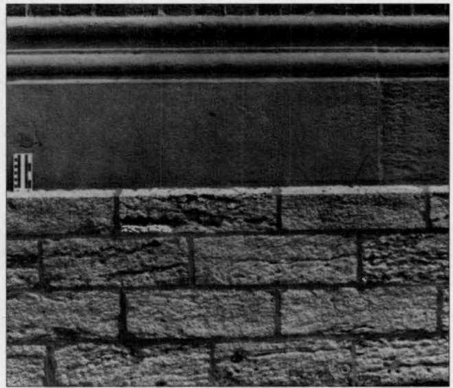
FIGURE 28.—Stone at the base of the Plum Street Temple. The lighter colored stone laid in courses is from the Fairview Formation ( Cincinnati limestone ); the darker stone above is fine-grained sandstone ( Buena Vista stone ). Photo taken in 1992.
