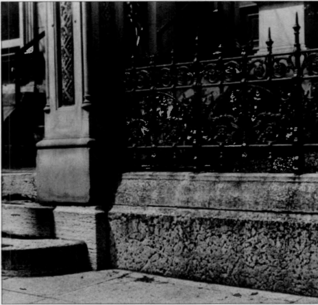
FIGURE 5.—Examples of some stone types that were widely used in the Cincinnati area in the mid-1800's can be seen in the older portion of Butterfield Senior Center, once the Cuvier Press Club. This building was constructed in 1862. The blocks of stone in the foreground are Dayton limestone . Note the wavy nature of the bedding of the blocks used for steps. Also note the elongate burrows seen in top or bottom view on the stone to the right. The pillar is fine-grained Buena Vista sandstone .
