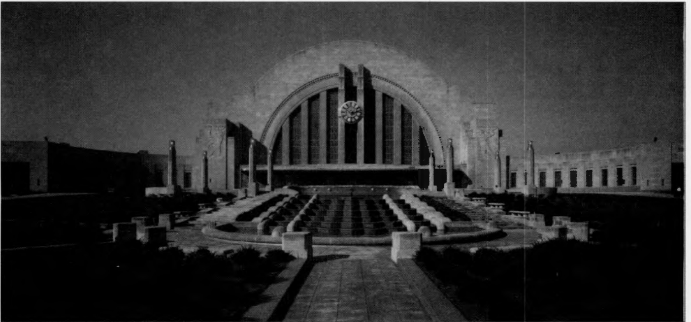
FIGURE 36.—Union Terminal (Museum Center). Photograph, taken in 1991, courtesy of The Museum Center at Cincinnati Union Terminal.
