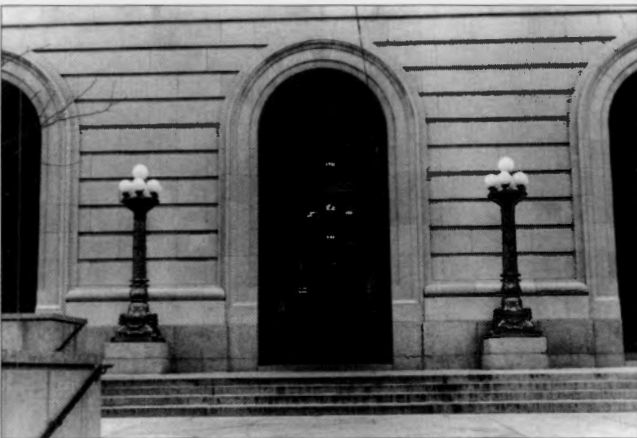
FIGURE 17.—West entranceway of the Hamilton County Courthouse. Photo taken in 1992.
