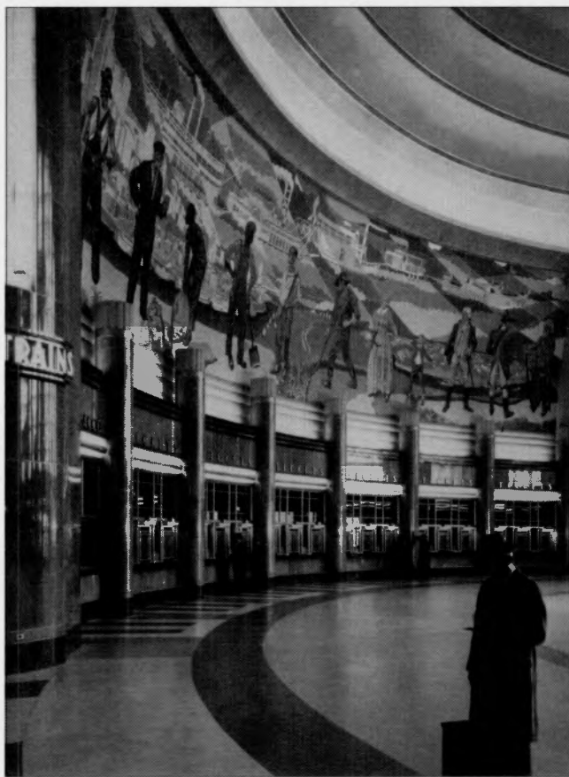
FIGURE 38.—Rotunda of Union Terminal. Photograph, taken ca. 1933, courtesy of The Cincinnati Historical Society.
