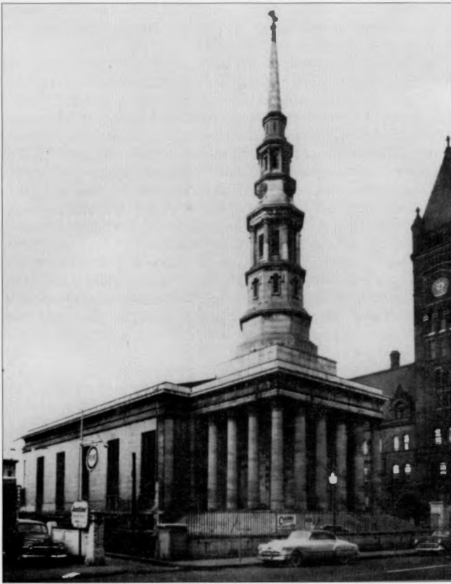
FIGURE 23.—St. Peter in Chains Cathedral, ca. 1950. City Hall is in the background to the right. Photograph courtesy of Hummel Industries, Inc.
