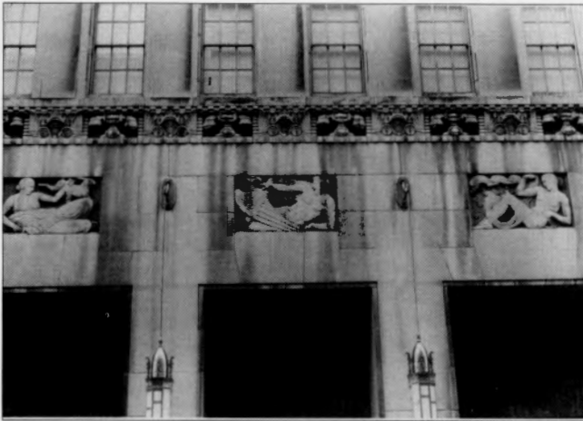
FIGURE 29.—Cincinnati and Suburban Bell Telephone Building. Note carvings (of Salem Limestone) of telephones under the windows. Photo taken in 1992.
