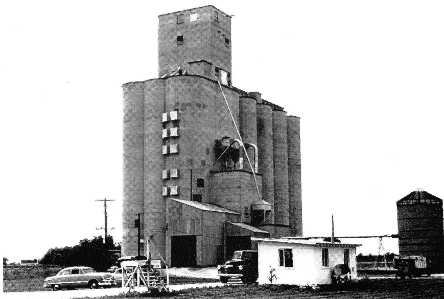
Fig. 9.—Dryer installed within the elevator. Notice the metal air exhaust vents on side of one of the silos.
