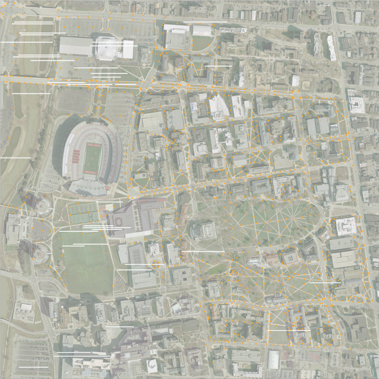
Each orange dot represents a street light’s location on main campus. Courtesy of ENGIE.
