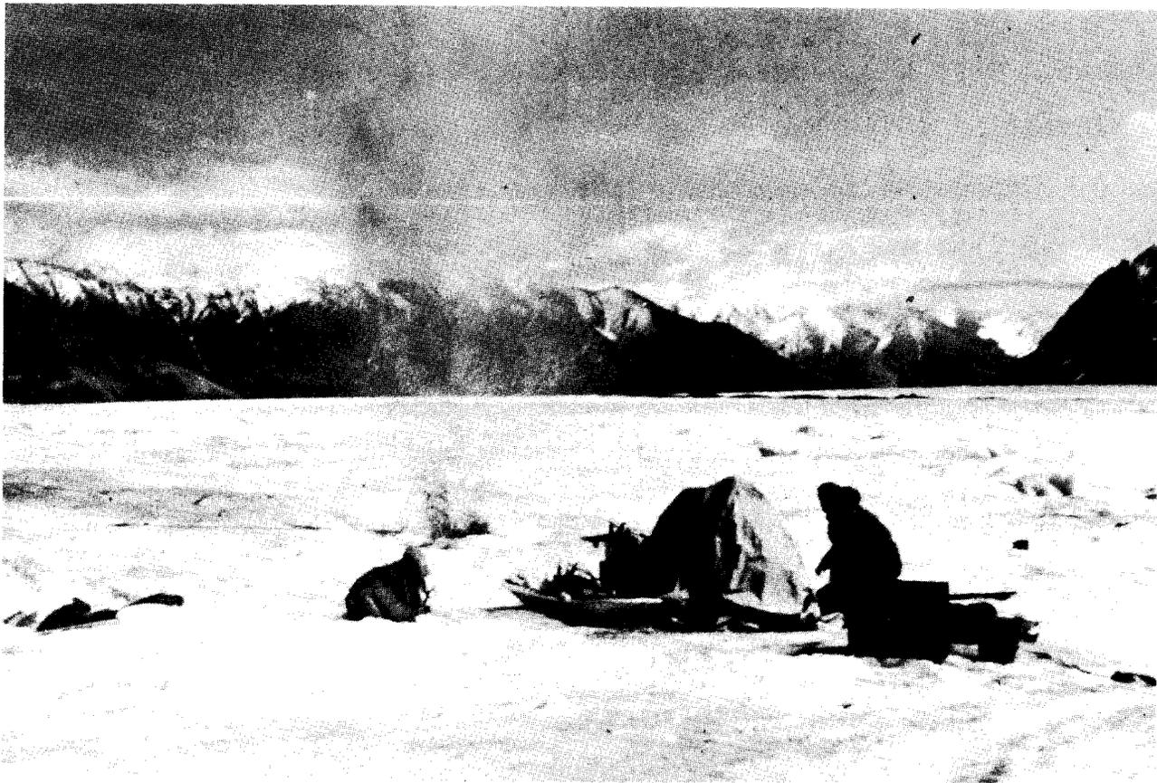
Figure 40. Seismic shooting on the Kaskawulsh Glacier.
