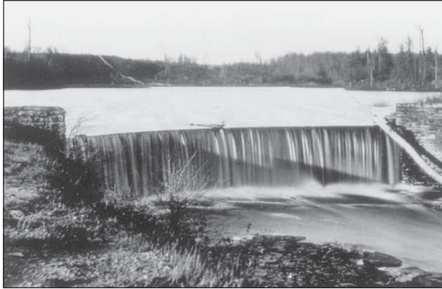
FIGURE 8-1.—Oldest available photograph of the IVEX Dam (circa 1870) showing the masonry spillway attached to bedrock on the west bank (left) and to an earth-fill dam on the east bank (right). The spillway was 7.4 m tall. Photo courtesy of the Chagrin Falls Historical Society.
