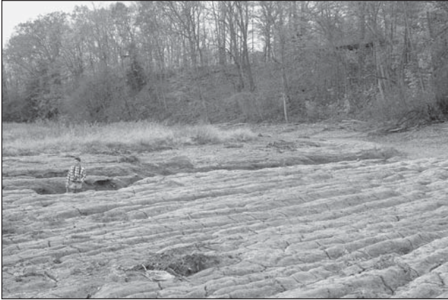
FIGURE 8-4.—Longitudinal scours in the reservoir sediment produced during the dam breach. Photo by J. Evans.
