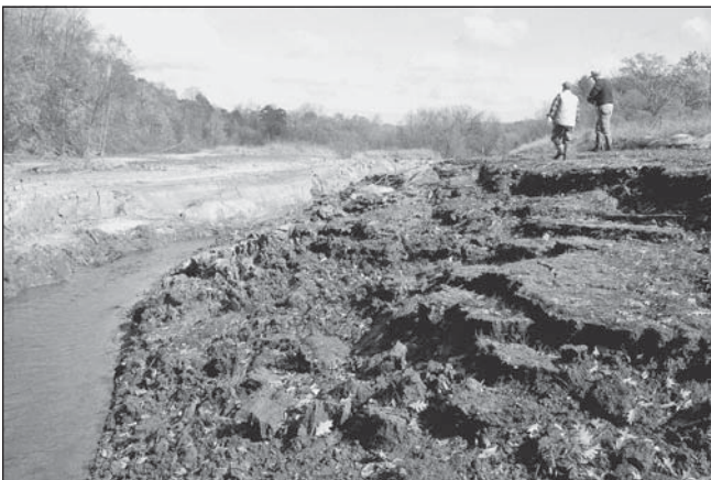
FIGURE 8-5.—Channel incision and slumping of reservoir sediments immediately following the dam failure, as the Chagrin River restores its channel shape and slope to the breaching of the dam. Photo by J. Evans.
