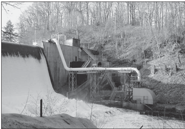
FIGURE 7-4.—Universal Electric Power's hydroelectric generator installed at the Ohio Edison Dam in Gorge Metro Park. Photo by A. Foos.
