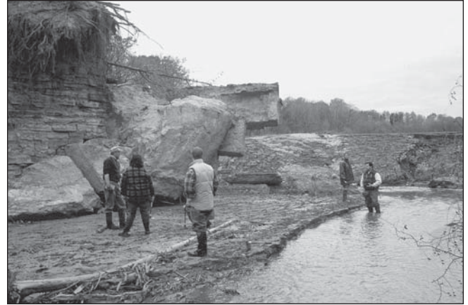
FIGURE 8-3.—Photograph of the breach in the dam taken several days after failure. The view upstream shows the approximately 4.5 m of sediment accumulated behind the dam. The lighter area on the spillway is a hydraulic cement patch from the 1985 partial seepage piping failure. Photo by J. Evans.
