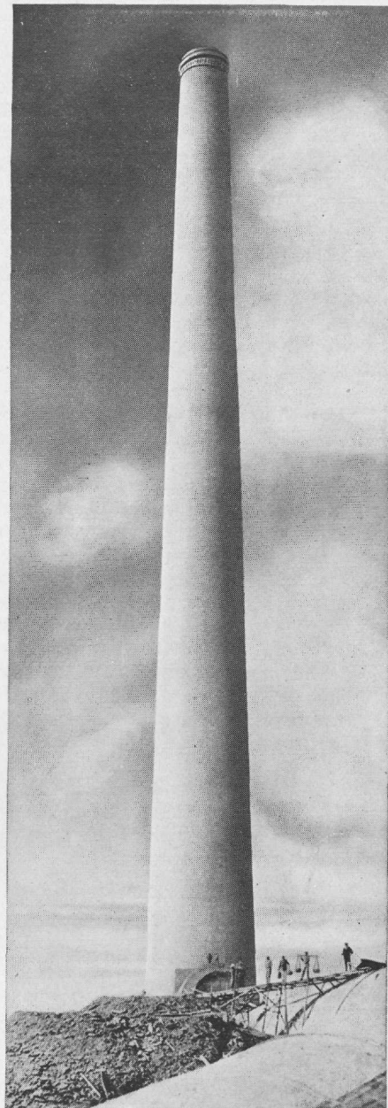
The Tallest Chimney in the World A 570-foot stack of the Saganoseki Copper Co., Saganoseki, Japan. Has withstood several violent earthquakes.
