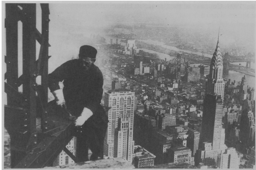
Lewis Hine's unconventional and humane view of New York's real estate boom included this photograph of a construction worker on the Empire State Building. The skyscraper was completed in 1930. Courtesy of the National Archives (American City List, #79, 69-RH-4K-1).
