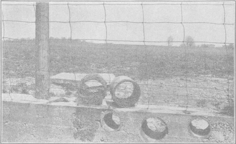
Fig. 11. Eight-inch tile one-third full of iron concretions.
