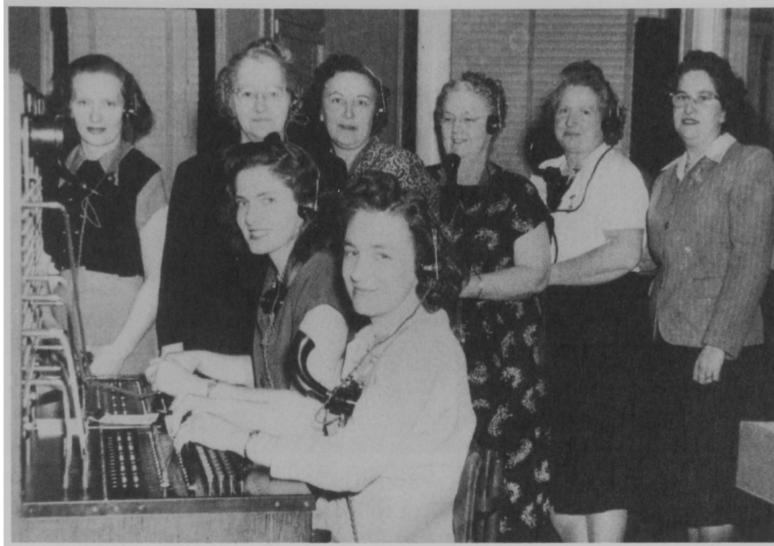
The communications center of American small towns was the local telephone switchboard. It remained part of Camden's life until the installation of modern switching equipment in 1959. The women who commanded Camden's switchboard posed for this picture in 1948. Courtesy Camden Archives.
