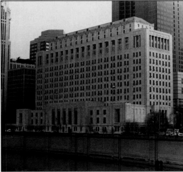
FIGURE 20.—Departments of State Building at 65 South Front Street. The Scioto River is in the foreground. In the background, the Riffe Center is on the far right next to the Huntington Center; at far left is the LeVeque Tower.
