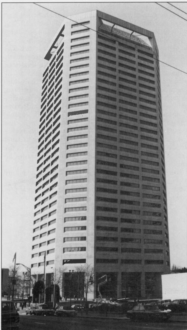
FIGURE 16.—American Electric Power Building.
