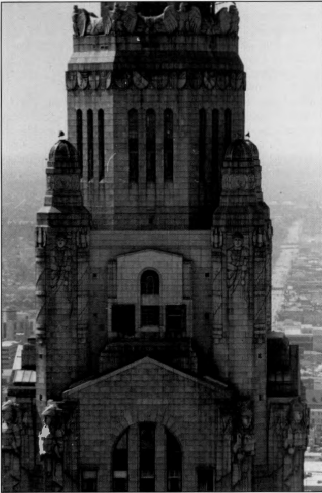
FIGURE 19.— Detail of terra-cotta sculptures on east side of LeVeque Tower. View from Rhodes Tower, 1986.
