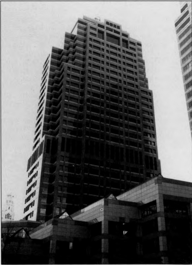
FIGURE 13.—William Green Building. The Atrium is in the foreground and Three Nationwide Plaza is on the right.
