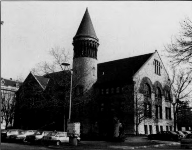
FIGURE 25.—Orton Hall at The Ohio State University. Five different Ohio building stones, arranged in stratigraphic order, were used on the exterior.
