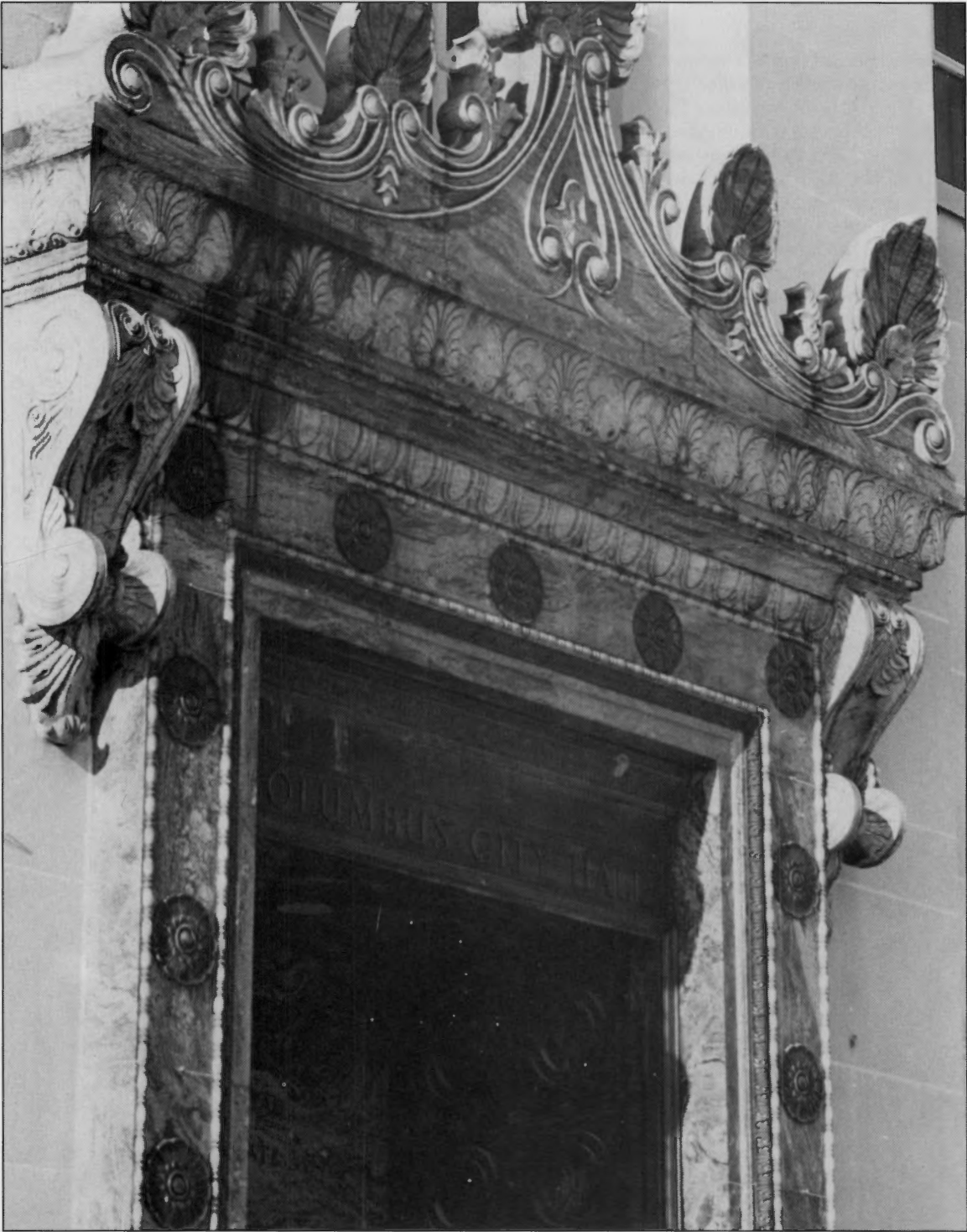
FIGURE 18.— Doorway of Morton Gneiss at Columbus City Hall.
