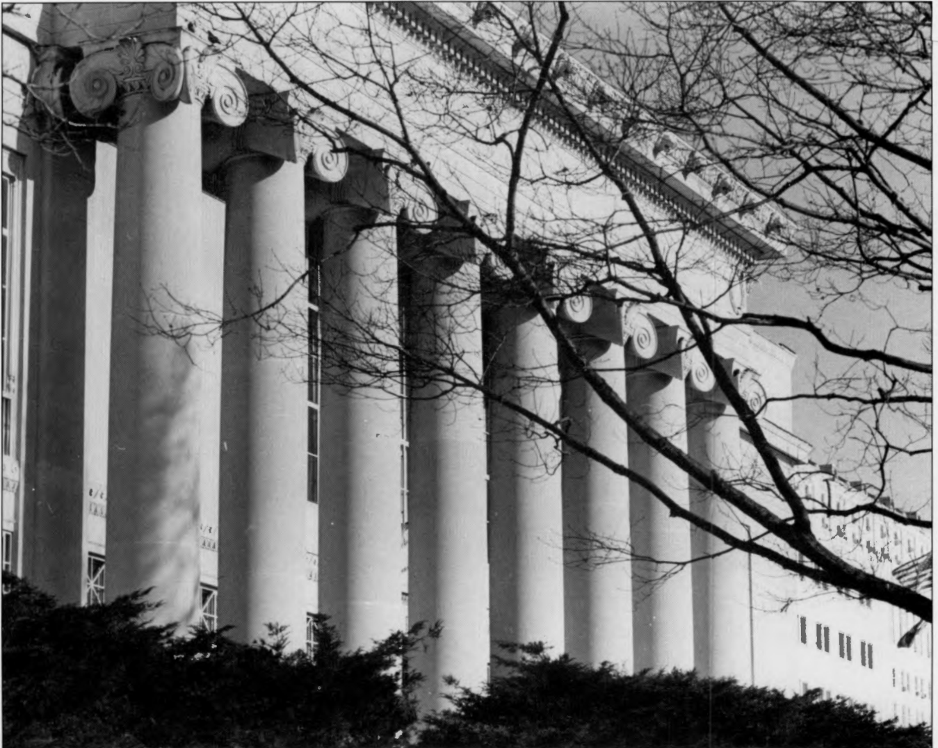
FIGURE 17.— Ionic columns of Salem Limestone on west side of Columbus City Hall.
