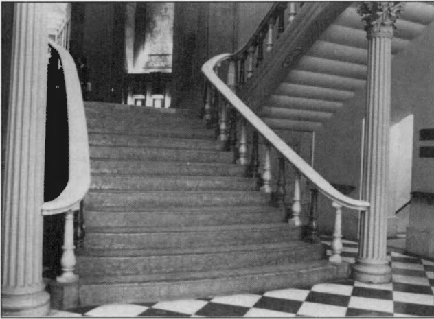
FIGURE 4.—Interior steps of Ohio State House showing stairs of Columbus Limestone, balustrades of Tennessee marble and white Italian marble , handrails of Italian marble , and floor of Champlain Black marble and white Italian marble .
