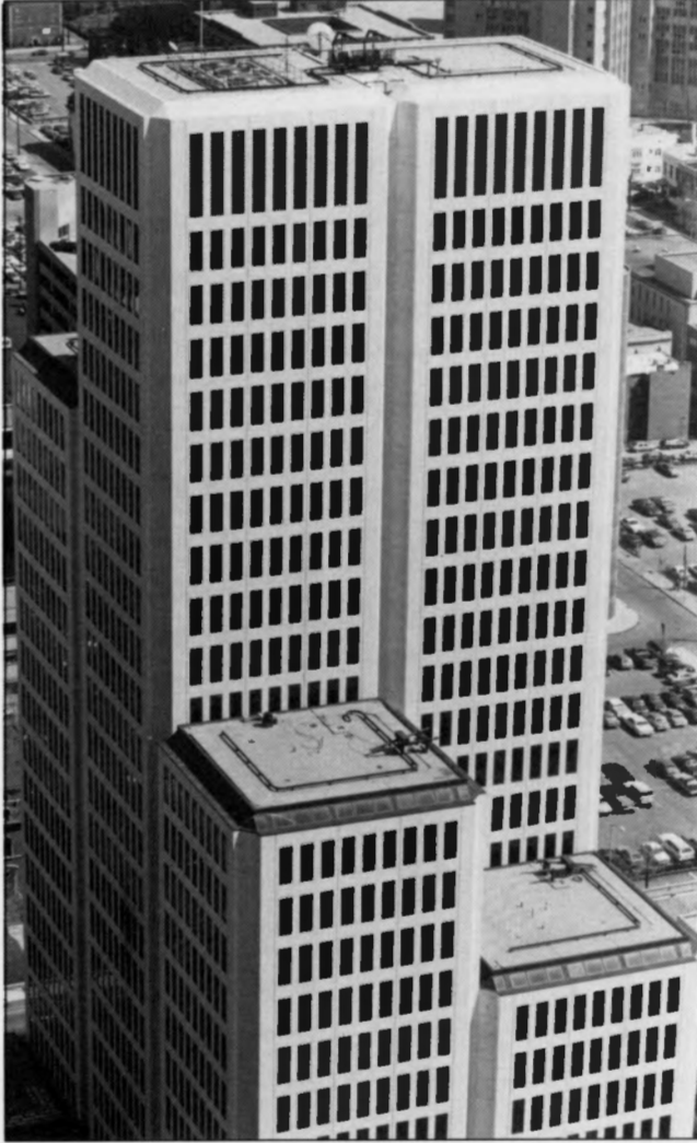
FIGURE 9.— BancOhio National Plaza. Five of the six connected towers are visible in this view east-southeast from the Rhodes Tower.
