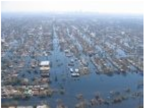
Views of inundated areas in New Orleans, Louisiana, following breaking of the levees surrounding the city as the result of Hurricane Katrina (2005).
