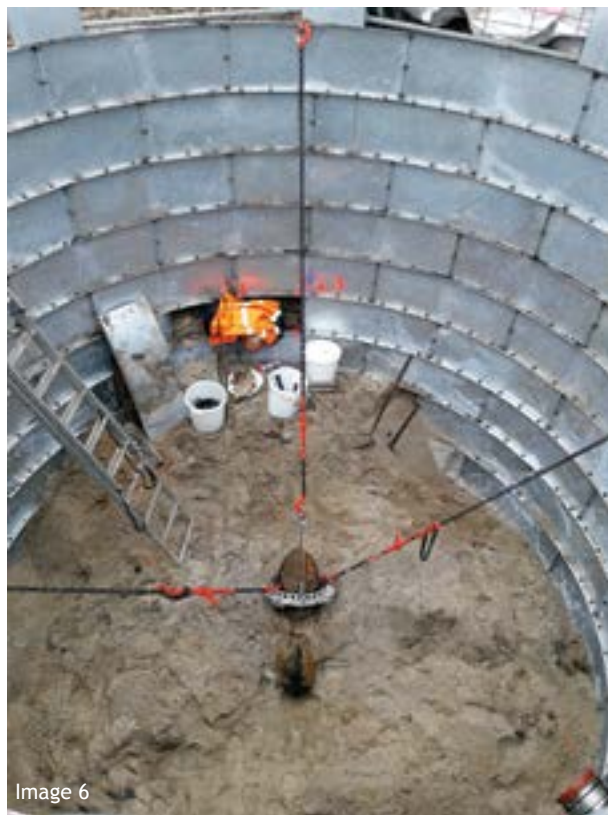
A 500 lb U.S. General Purpose (GP) bomb subsequently excavated at this site. The target was reflected off of bedrock, resulting in a nose-up orientation that prevented triggering of the delayed-action fuse.
