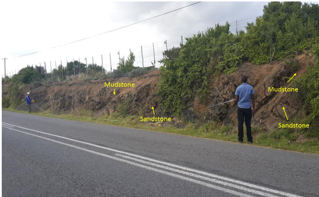
Figure 3.27: Photograph showing grey mudstones alternating with minor sandstones along National road N2 between Grahamstown and Peddie.
