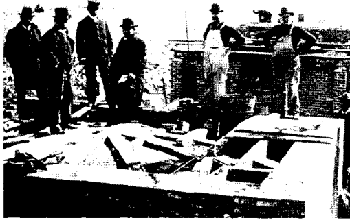
Figure 3 Fire-resistance test with a timber vault (New York, 1897). (Guastavino is the second from the left)
