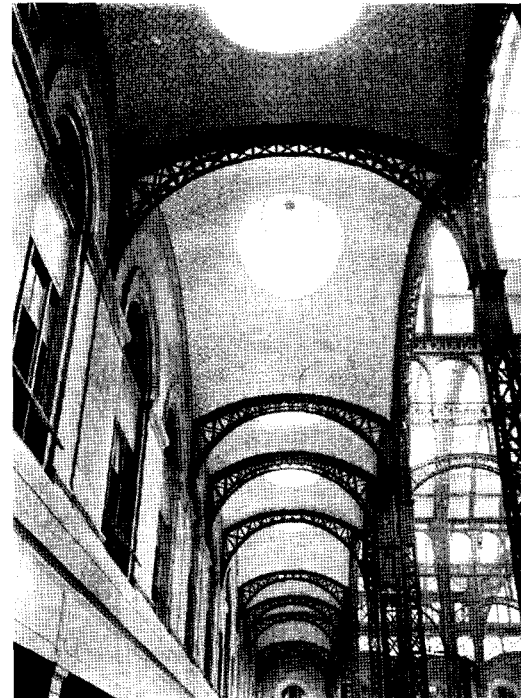
Figure 4 Pennsylvania Station, New York, 1905–1909. (Demolished in 1963). (With McKim, Mead & White)
