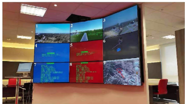
Figure 12. Video Wall Implementation
