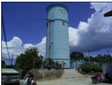
Distribution has improved markedly since privatisation with rehabilitation of network and storage facilities such as this BWUI water tower.
