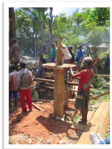
Figure 1.13a–c: Men install the first pillar, ( sa'a , M) of the oma falu at Bubuha, Larisula, Baguia Sub-district, 16 August 2014. The installation of this pillar is part of the dada sa'a and sa'a falu phases of building an oma falu .
