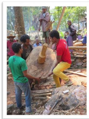
Figure 1.13a–c: Men install the first pillar, ( sa'a , M) of the oma falu at Bubuha, Larisula, Baguia Sub-district, 16 August 2014. The installation of this pillar is part of the dada sa'a and sa'a falu phases of building an oma falu .
