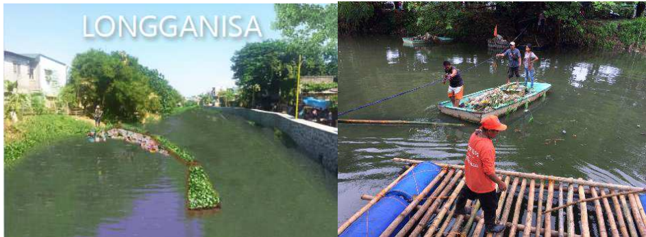
Fig. 8. Design of innovative ‘Longganisa’ to remove floating waste from rivers. 9b: the Longganisa constructed November 2016 (in the back is the old way of collecting trash from the river with a boat).
