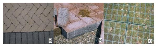
Figure 1 (a) Impermeable Concrete PICP; (b) Porous Concrete PICPs; (c) Grass-filled PICPs.
