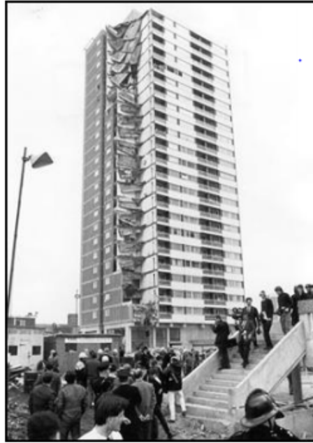
Figure A.1 : Ronan Point After Collapse
