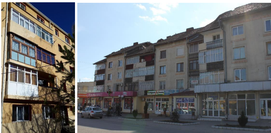
Fig. 4.26: Interventions over facades for block 'N' (left) and 'A' (right).
