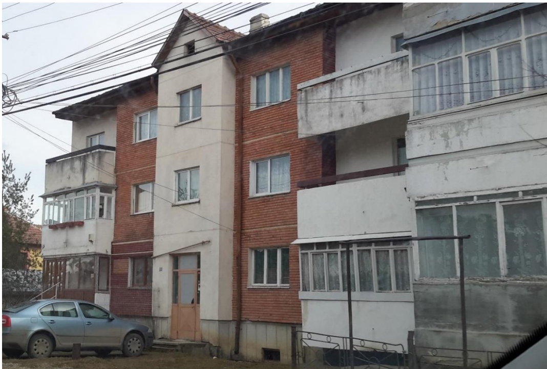
Figure 4.27: Interventions over facades for block ‘D’ (above) and block ‘J’ (below).
