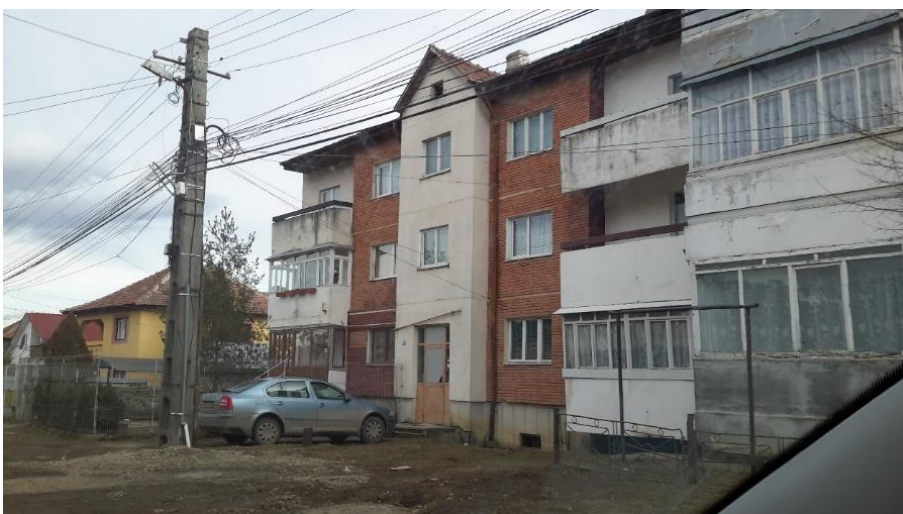
Figure 3.15: Block ‘J’ situated in the secondary center near Refinery.
