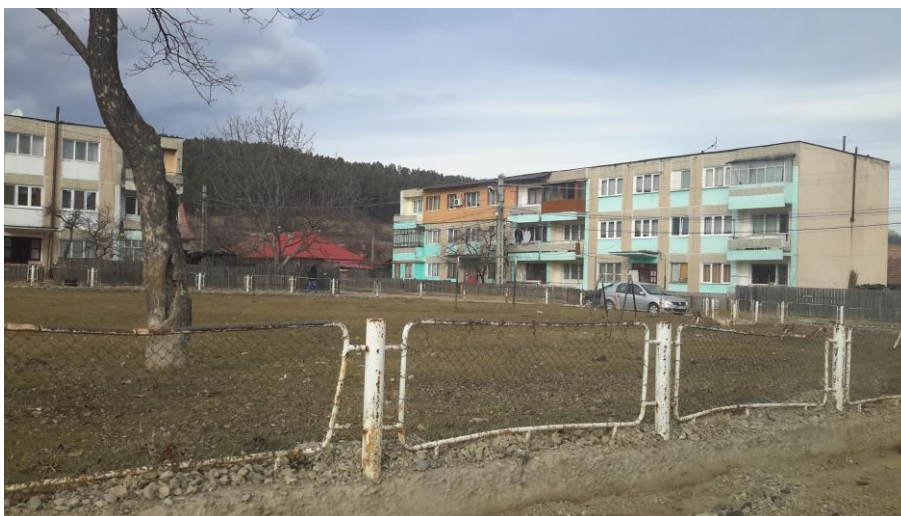
Figure 3.12: Block 'D' situated in the secondary center near Refinery.
