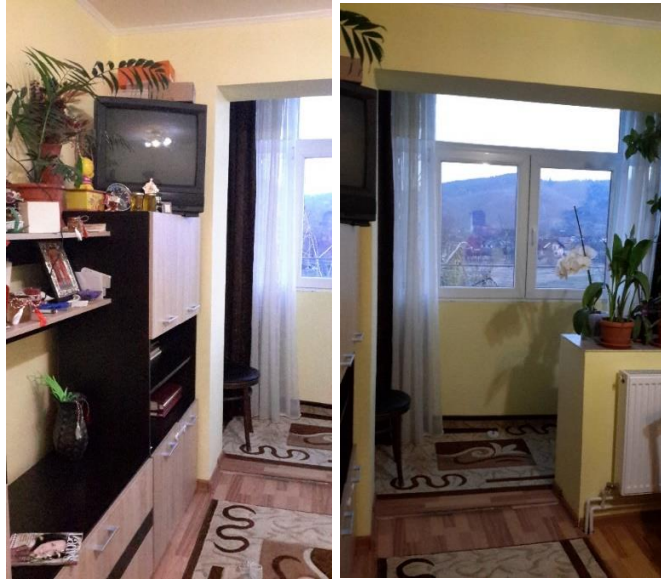
Figure 4.19: Extension of the living room and the reconstruction of walls for the balcony in F11 .
