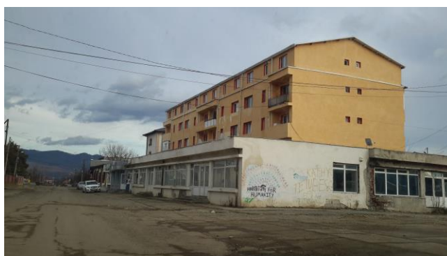
Figure 3.17: Block 'N' situated in the secondary center near Refinery.
