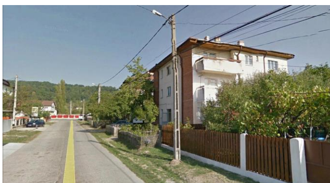
Figure 3.19: Blocks 'L' and 'M' situated in the secondary center near Refinery.
