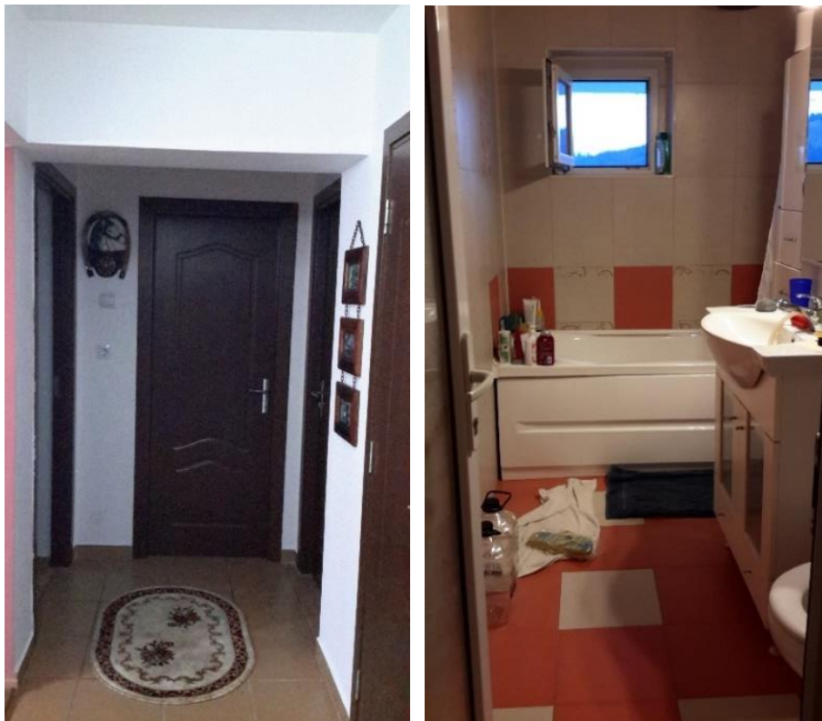
Figure 4.32: Example of floor renewal in F1 (left) and F8 (right).
