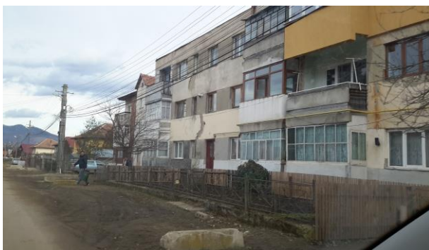
Figure 3.16: Block 'K' situated in the secondary center near Refinery.
