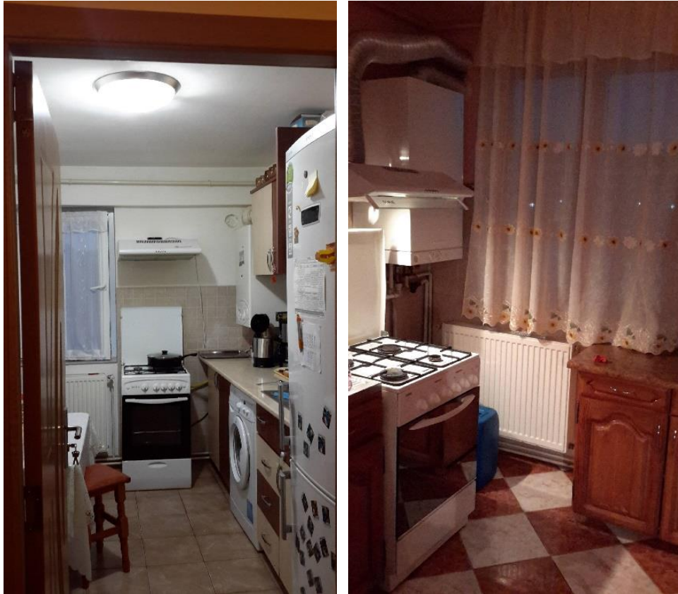
Figure 4.33: Example of floor renewal in F11 (left) and F2 (right).
