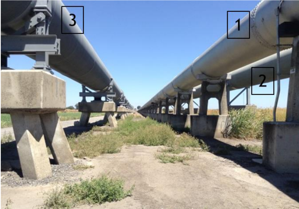
Figure 4. Mokelumne Aqueduct, Sacramento-San Joaquin Delta, California. June, 2017. Aqueducts No. 1, No. 2, and No. 3.
