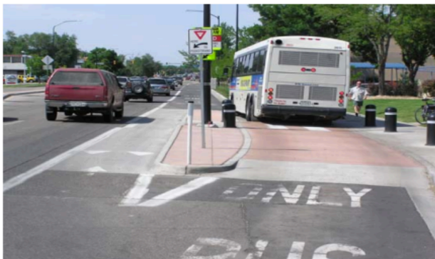
Fig 4: Bus stop designed to leave room for cyclists in Boulder, CO. Source: City of San Jose, 6-3, 2009.
