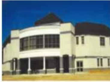
r) PM building, USA (Biggs, 2003)
