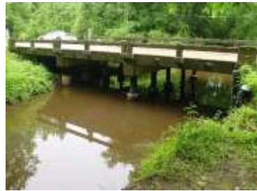
b) Vehicular bridge (Wight, 2006)
