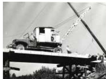
aa) Vehicular bridge, Tennessee, USA (Bennett, 2008)
