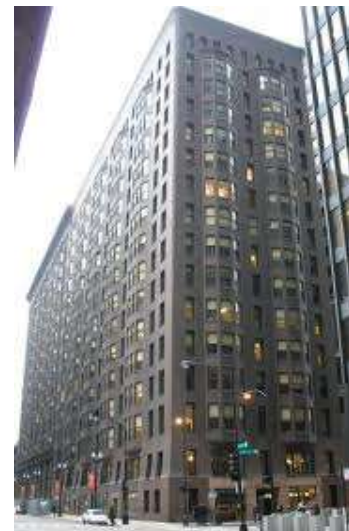
Figure 2. 1 Monadnock Masonry Building, Chicago (Ganz, 1990).
