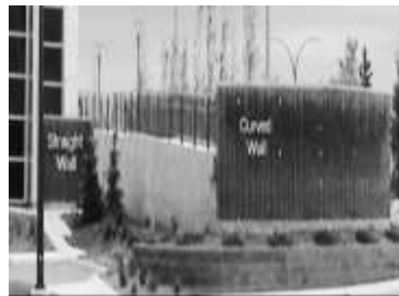
f) Retaining wall U. of Calgary (Lissel et al., 2005)
