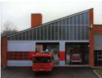
e) Rushden Fire Station, (Allen, 1986)
