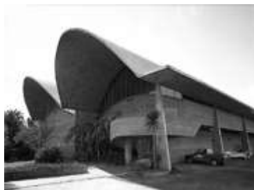
ad) Industrial building, Refresco del Norte, Salto Uruguay (Pedreschi, 2004).
