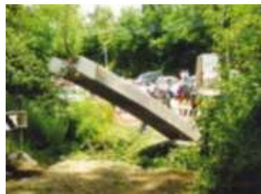
j) Pedestrian Bridge, (Ganz, 2003)
