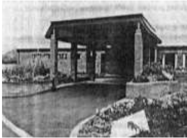
q) Ambulance Garage Columns (Shaw, 1988)
