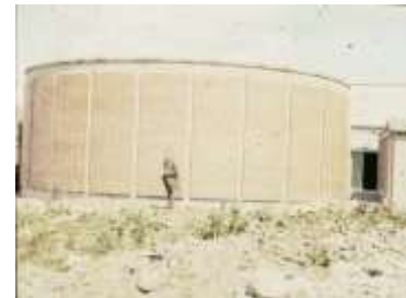
x) Prestressed circular water tank (Sinha, 2002)
