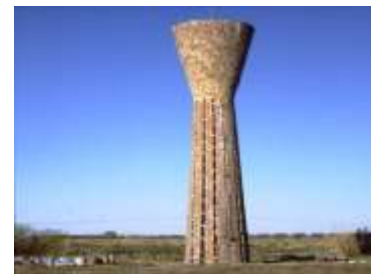
af) Masonry water tower, Uruguay (Sinha, 2002).
