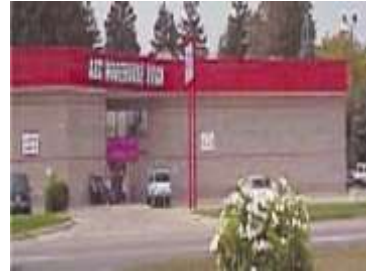
s) Supermarket repaired with PM (Biggs, 2003)
