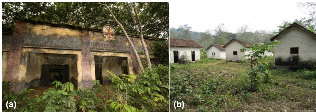
Fig. 1 (a) Abandoned hospital and (b) workers' houses near Tchilumbo village. All these infrastructures belonged to the Angolan Company of Agriculture in Amboim (CADA Amboim) – photos taken by A. Estrelinha and M. Mills respectively
