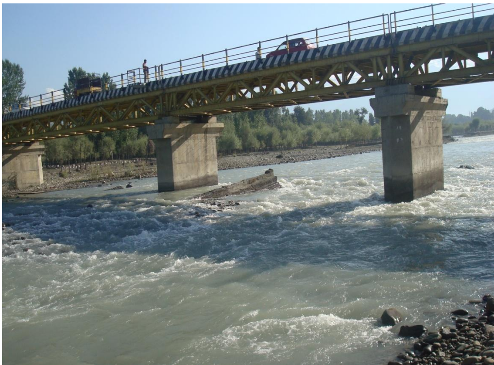
Phg-2: A view of Lidder Stream at Site-II
