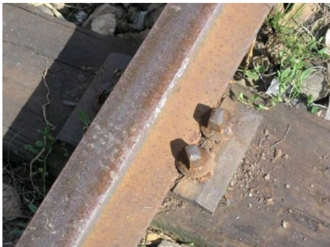
Fig. 8.1 An example of a direct, rigid fastening of rails to the wooden sleepers ( http://www.transportszynowy.pl/kolprzytw1bezp.jpg )
