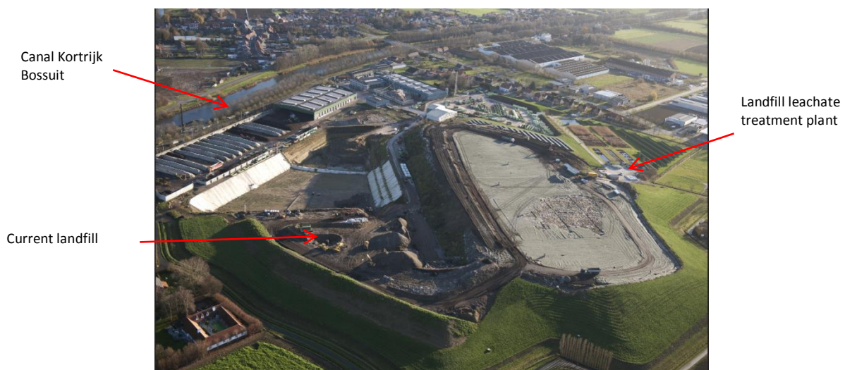
Figure 3.1: Birds eye view on the IMOG landfilling facility.
