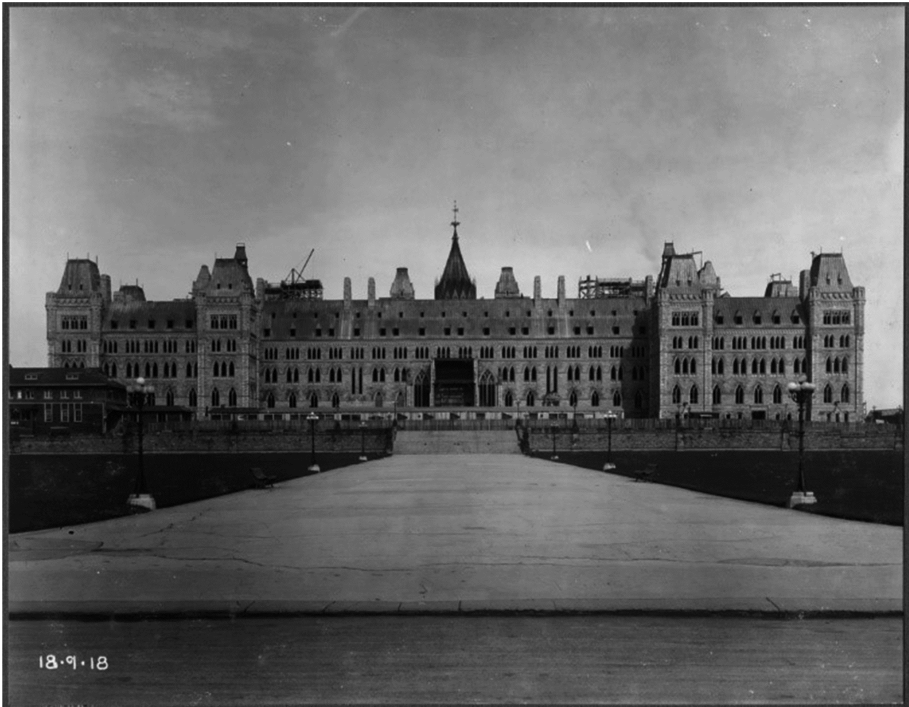
Fig. 1. Historical Picture of the Centre Block under construction. Date: 1918-09-18 Source: Library and Archives Canada, Image#e010865984
